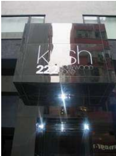
Old 222 canopy with signage
