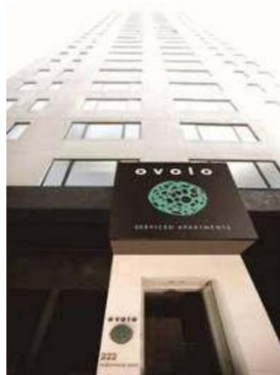
Transformed 222 canopy with signage
